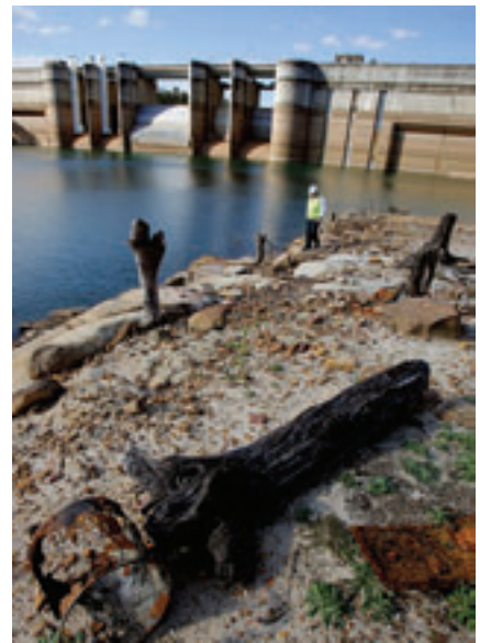
Sydney's Warragamba Dam, September 2004, at its lowest level ever—just 39.9 percent capacity. With the state of New South Wales already in the grip of a severe drought, the city of Sydney is currently experiencing its longest drought since the 1930s, and with the population growing at an average of 50,000 per year, it is putting an enormous pressure on the dwindling water supply. With tight restriction on water usage already in place, the government is being pressured to implement even tougher rules, with some reports suggesting the city's water supply may run out in just over three years.
